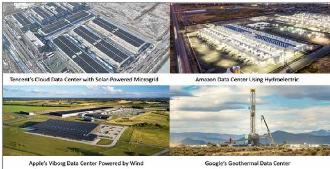
Figure 2. Sample OT environments (data centers) with upgraded energy support systems
